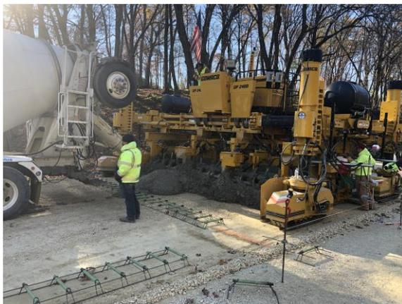
*The paving machine is set up to pave one half of the road at a time which in this section is 20 feet wide (photo courtesy of McClure Engineering).*
