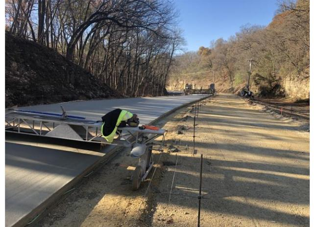
*After the paver places the concrete, finish work follows close behind. This includes application of curing compound, grooving, and cutting joints (photo courtesy of McClure Engineering).*
