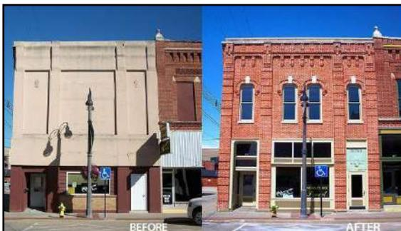
**Left, *BEFORE* photo: A building whose brick facade was covered with a masonry-type material in the past. This may have been done to modernize its appearance or to attempt to protect the brick.**
